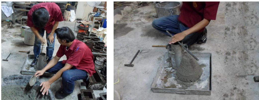
Figure 3. Slump test of concrete
